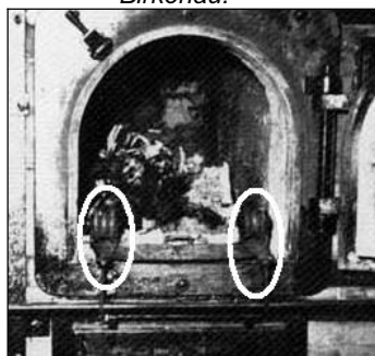
III. 135: Rollers in front of the muffle to insert the stretcher (highlighted with white ellipses). 1179
