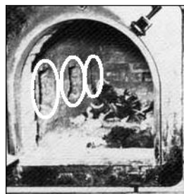
III. 137: Openings in walls of center muffle of Buchenwald triple-muffle oven (=Birkenau ovens, highlighted with white ellipses). 1179
