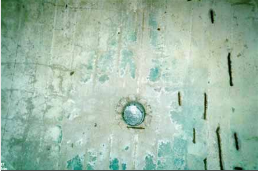
Photo 10: Delousing chamber in Stutthof, interior. Circular opening in the middle of the reinforced concrete ceiling; note the typical blue pigmentation due to iron cyanide. The opening was used for the introduction of Zyklon B into the delousing chamber. © Carlo Mattogno
