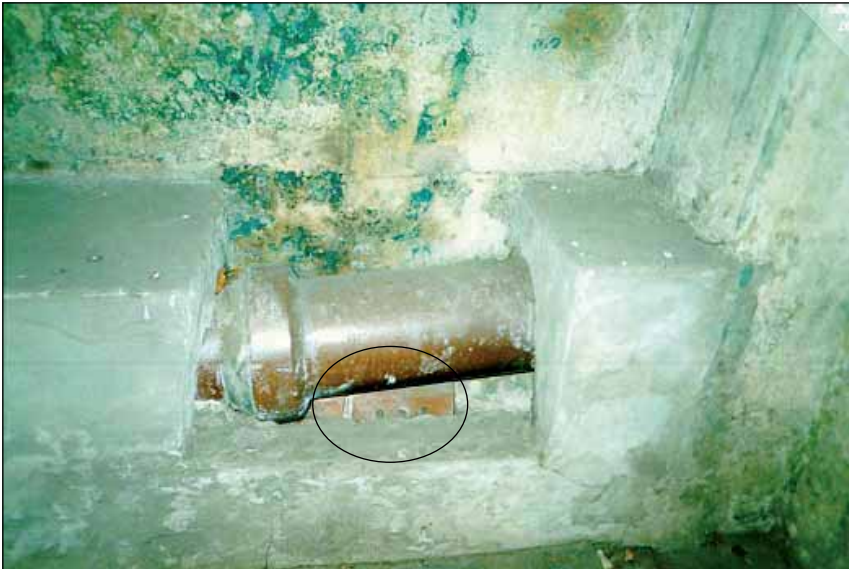
Photo 8: Delousing chamber in Stutthof, interior, west wall; cast iron connection pipe to the oven installed outside the gas chamber, which was used to heat the air. The pipe was originally surrounded by masonry, similar to that visible in the photo, but perforated. One of the perforated bricks is still visible below the pipe (circle). © Carlo Mattogno
