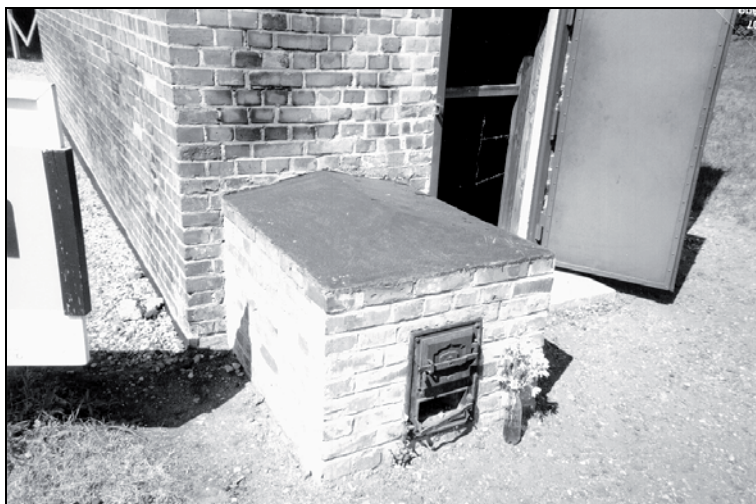
Photo 5: Delousing chamber at Stutthof, viewed from the south. The oven was used to heat the air inside the delousing chamber. © Carlo Mattogno
