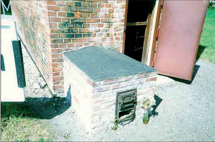
Photo 5: Delousing chamber in Stutthof, south side. Oven to heat the air in the gas chamber. © Carlo Mattogno
