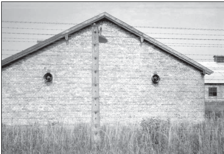
1. Birkenau, BW 5b, round openings for placement of ventilators in the outside wall of the gas disinfestation chamber. July 1992, © Carlo Mattogno.
