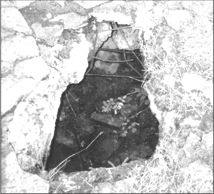
III. 17: Concrete roof of morgue 1 of crematorium II in Birkenau. Provan's opening 2 in July 1992. © Carlo Mattogno
