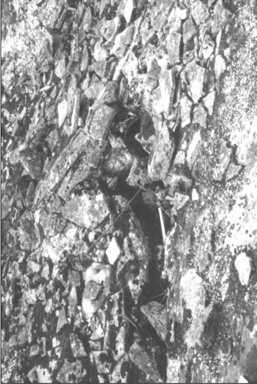
III. 31: Concrete roof of morgue 1 of crematorium II in Birkenau. Provan's opening no. 6 in August 2000. © Carlo Mattogno
