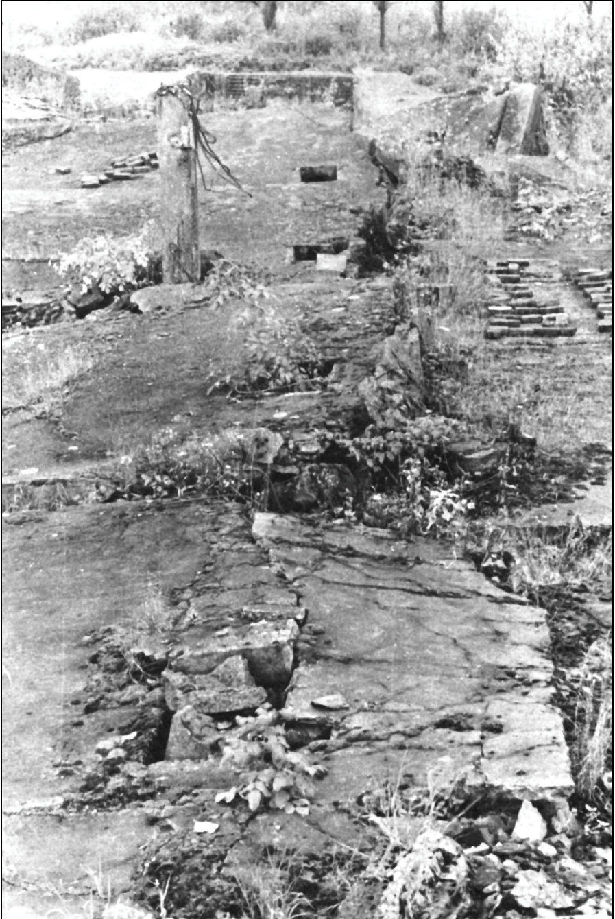
III. 14: All five ventilation openings of the ceiling of the oven room of crematorium III. Photo by J.-C. Pressac.
