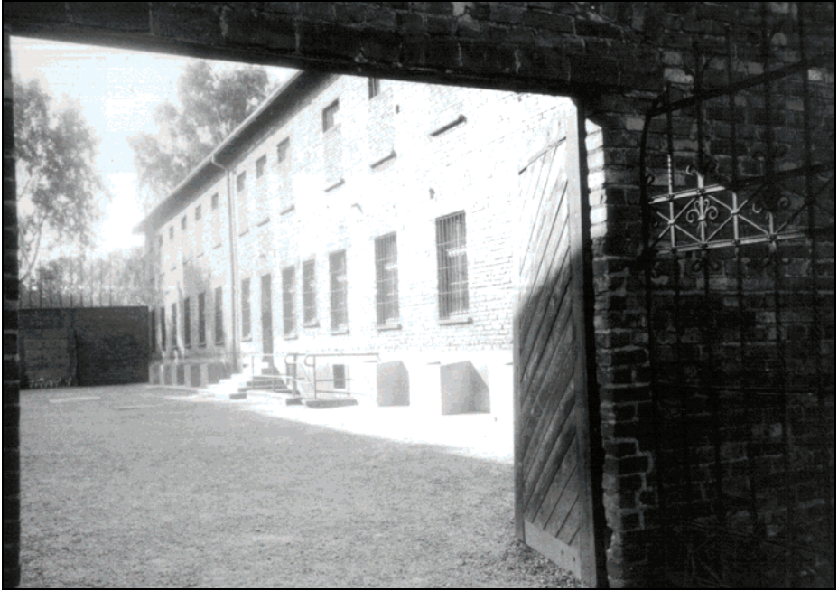
Photo 2: Block 11, outside, wall facing NNE, yard. © Carlo Mattogno, Oct. 1991
