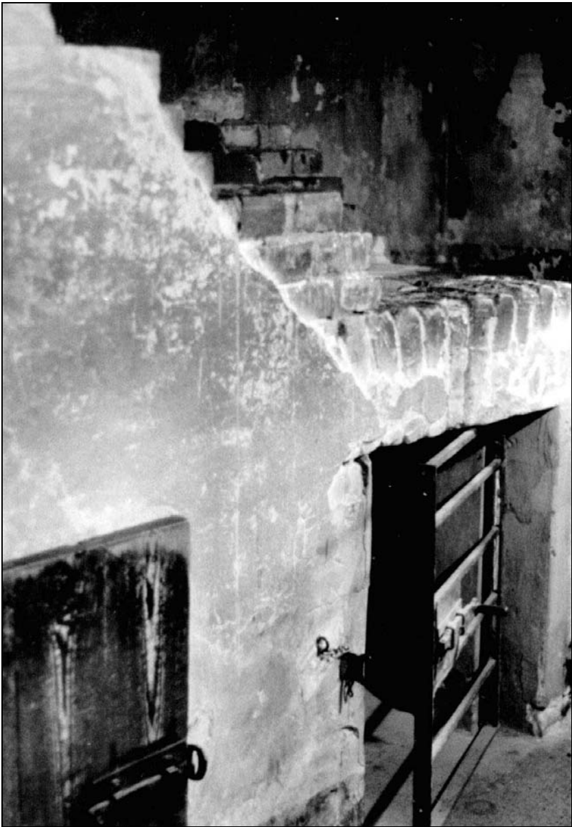
Photo 32: Block 11, inside, Bunker, right side, stand-up cells.
