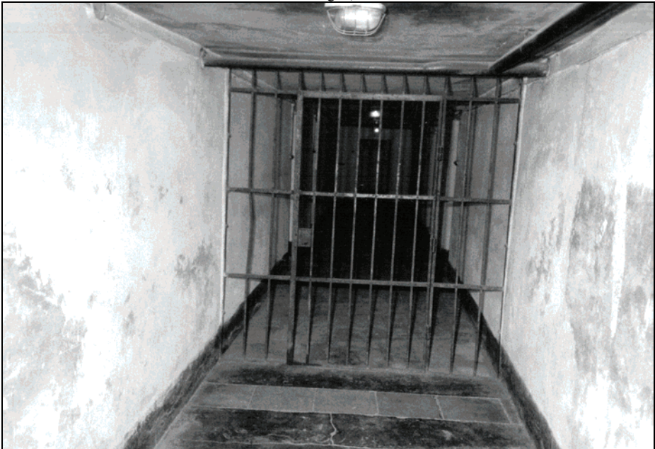
Photo 12: Block 11, inside, Bunker, iron grid separating the left side of the Bunker from its right side. © Carlo Mattogno, Oct. 1991
