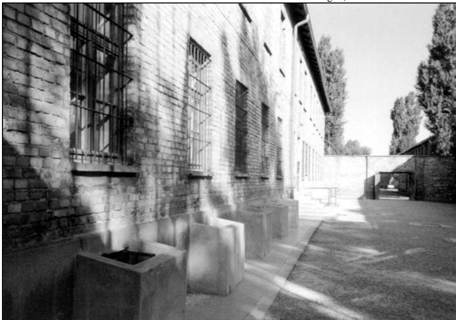
Photo 22: Block 11, outside, wall facing NNE, concrete covers surrounding the windows of the Bunker cells. © Carlo Mattogno, Oct. 1991
