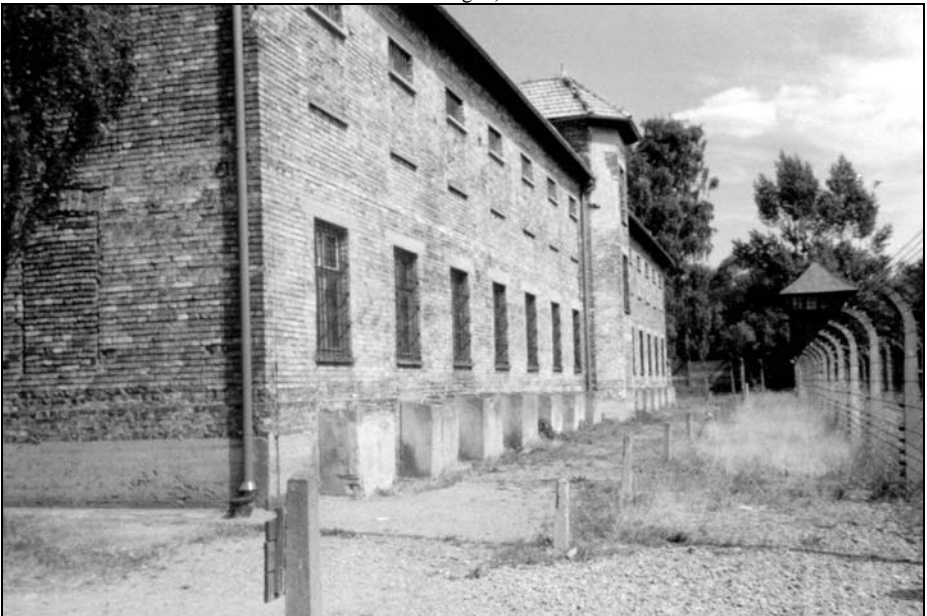
Photo 26: Block 11, outside, wall facing SSW, concrete covers surrounding the windows of the Bunker cells. © Carlo Mattogno, Oct. 1991
