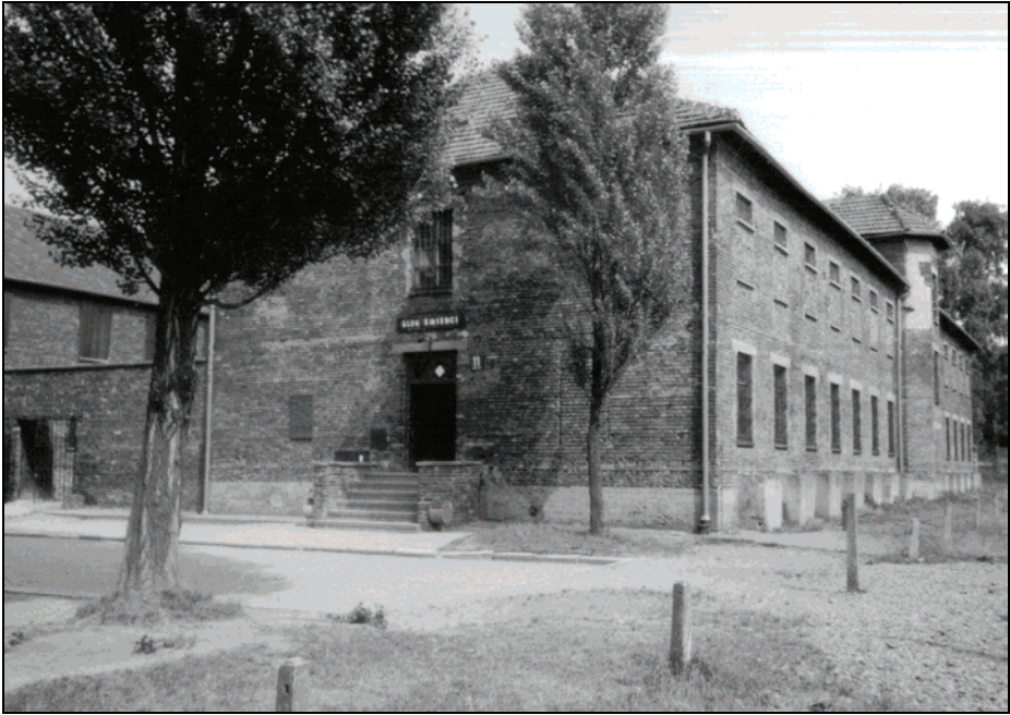
Photo 4: Block 11, outside, walls facing NE and SSW.
