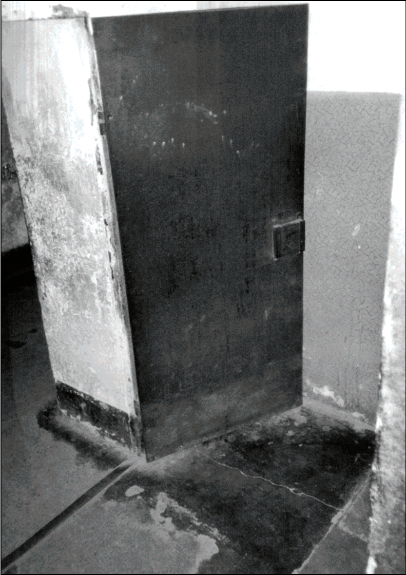
Photo 10: Block 11, inside, steel door of the Bunker seen from the stairs. © Carlo Mattogno, Oct. 1991
