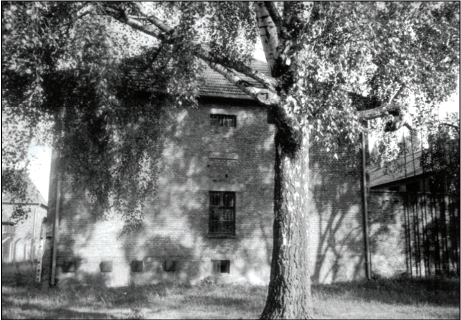
Photo 29: Block 11, outside, wall facing SE, sheet-metal boxes covering the air-supply holes of the 4 stand-up cells ( Stehzellen ) of the Bunker. In the center underneath the large window: window of cell no. 21 (see photo 17).
